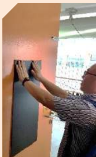
Mounting of the corrugated black-out board at the classroom door.
